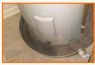
Make certain that it sits in a tray—in the event of a leak, water won't leak everywhere. You may want to have a plumber flush out the water heater to remove any minerals or dirt that settle at the bottom of the heater. This sediment in the water can eventually rust out the bottom of the heater. You should also ask the plumber if he thinks the heater anode needs replacing.
