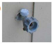
Turning it off inside is not enough. The water in the pipe could freeze and cause the pipe to burst inside your home. First, locate the turn off valve in your basement,
