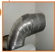
Don't forget to have it cleaned as well—a lint filled vent has been the source of many, many fires. And if your dirty dryer vent, vents to the attic and not outdoors, it could also is
