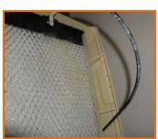
Humidifying system: Check the filter as well. It should be replaced annually, but consult the owner manual for model specifics and for the removal and cleaning of the filter assembly. No manual? Google your humidifier brand—it'll be online.
