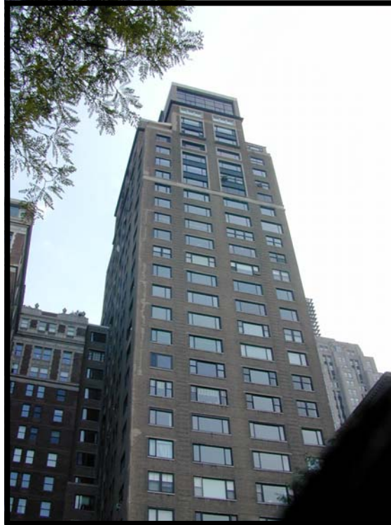
179 E Lake Shore Dr. (Drake Tower), Chicago, IL 66 unit cooperative built, 1928-31; Architect: Benjamin Marshall Benjamin Marshall;
