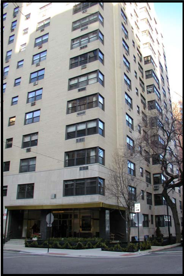
1335 N Astor, Chicago, IL, 31 unit, 16 story coop; built, 1926
